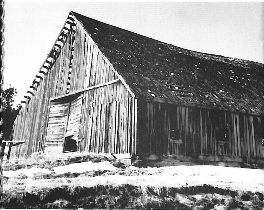
Remains of an old barn at a stage stop on Combs Flat along Steens Wagon Road.
