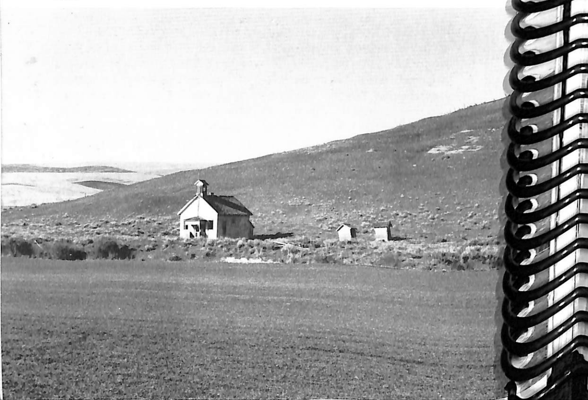
The Eightmile Schoolhouse south of The Dalles. The Barlow Road went by here.
